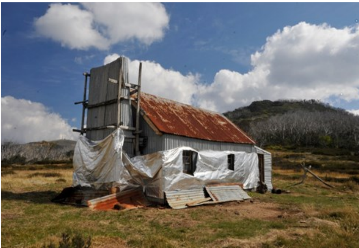
Spargo's Hut wrapped in aluminized and glass fabric to protect the building against radiant heat. Fortunately, the fires did not reach the locality and the building was spared again.
