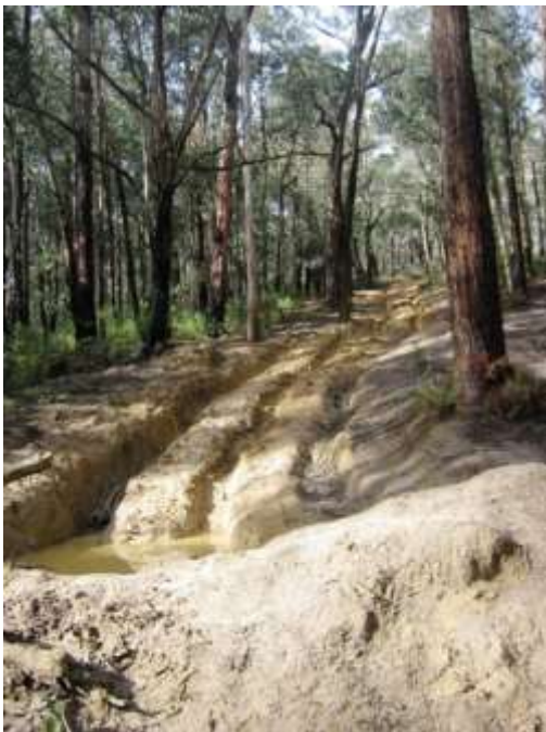
Damage done by 4WD going over a hump on a track
