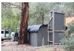
The renovated Store Point Hut, which survived the recent fires
